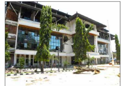
Figure 7. Padang city government buildings, including a collapsed 3-story building (left) and newer 4-story building (right) with extensive nonstructural damage.
