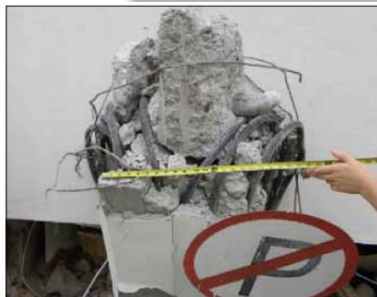
Figure 8. First-floor collapse in 3-story office of the Provincial West Sumatra Planning Building, constructed in 1983.
