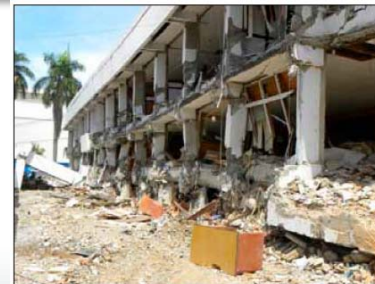
Figure 7. Padang city government buildings, including a collapsed 3-story building (left) and newer 4-story building (right) with extensive nonstructural damage.
