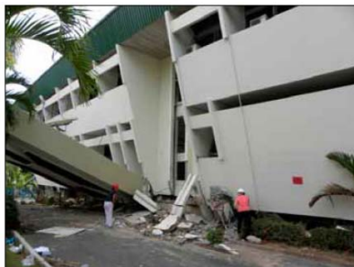
Figure 8. First-floor collapse in 3-story office of the Provincial West Sumatra Planning Building, constructed in 1983.
