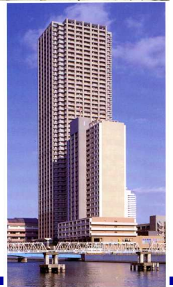
HARUMI Island Toriton-square-View-Tower
